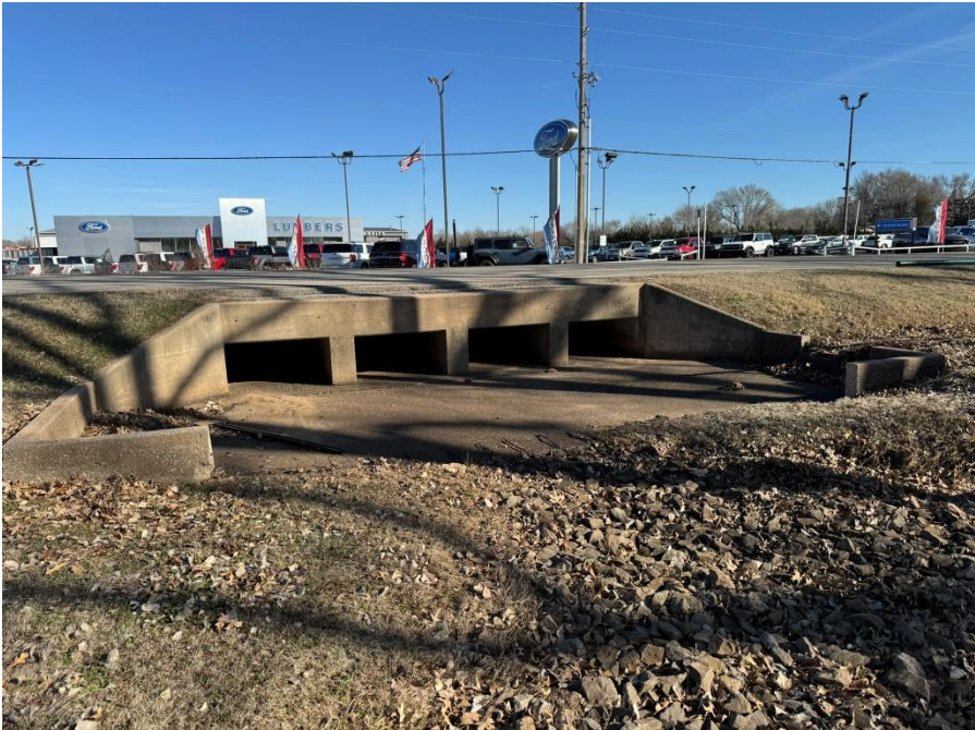
Figure 1 Upstream Cross Road Culvert
