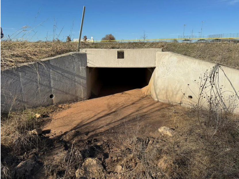
Figure 14 Downstream Culvert End
