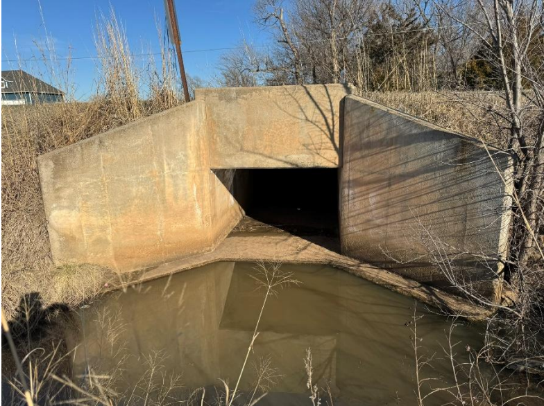
Figure 9 Upstream Culvert End
