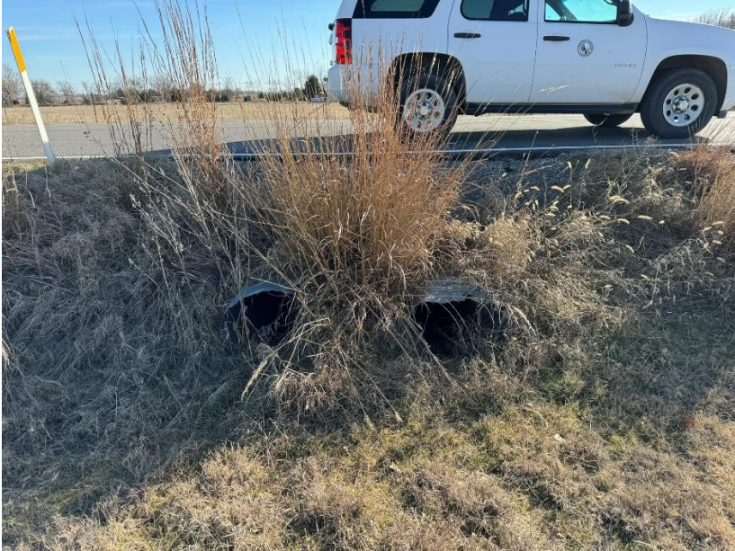
Figure 11 Upstream Culvert End
