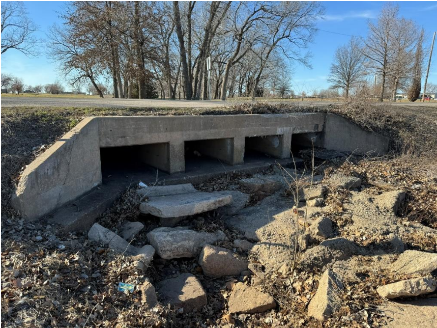
Figure 2 Downstream Cross Road Culvert
