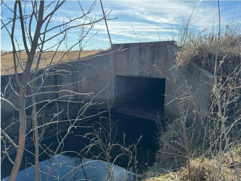
Figure 10 Downstream Culvert End
