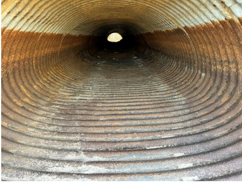
Figure 7 inside Culvert Condition
