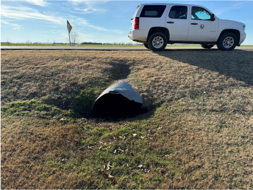
Figure 4 Downstream Culvert End
