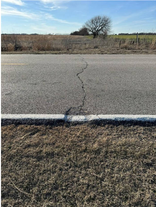
Figure 8 Road Condition over the South Cross Road Culvert
