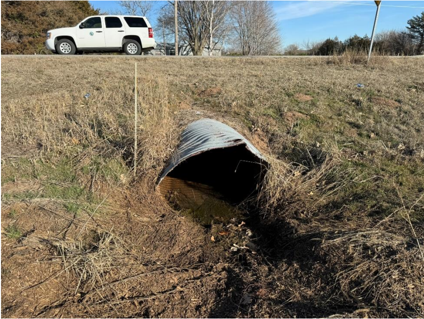
Figure 3 Upstream Culvert End
