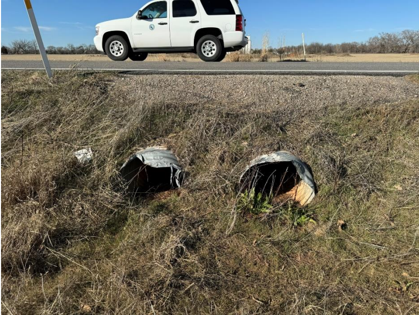
Figure 12 Downstream Culvert End
