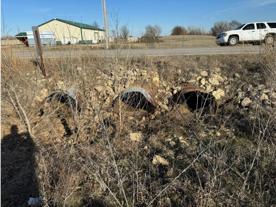
Figure 5 Upstream Culvert End
