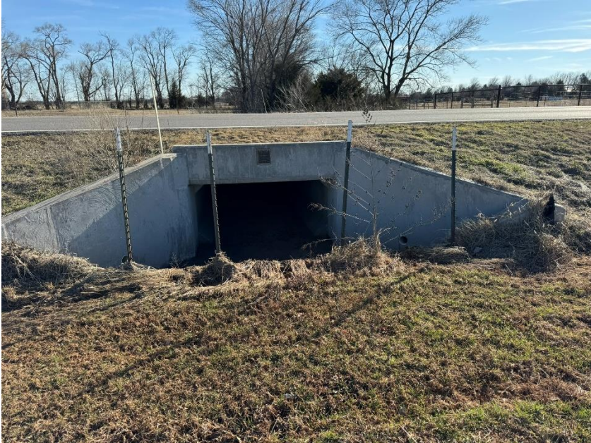
Figure 13 Upstream Culvert End
