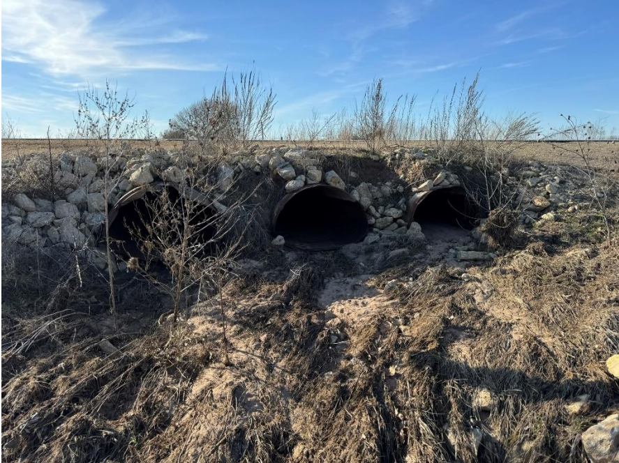
Figure 6 Downstream Culvert End
